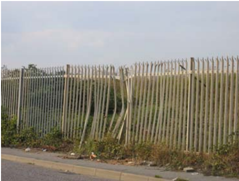
Old style industrial palisade fencing
